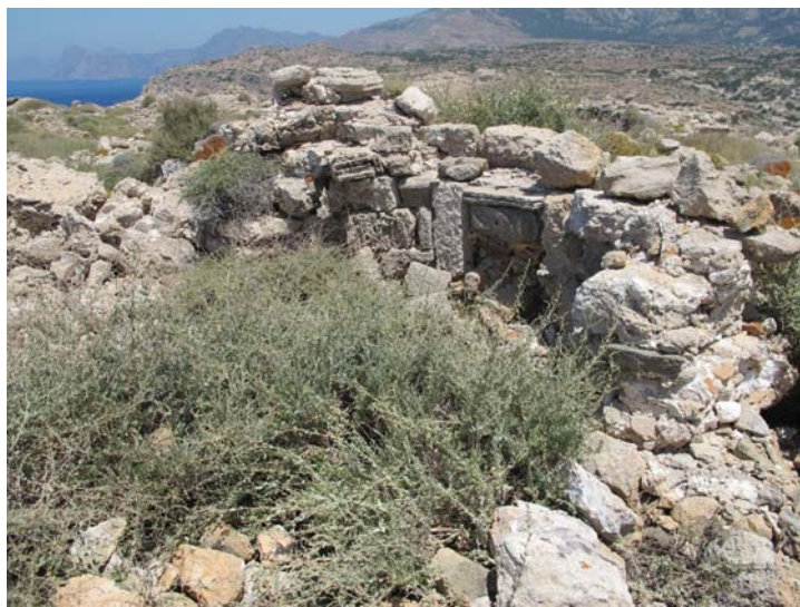
Figure 4: Niche in Apse wall, B1137
